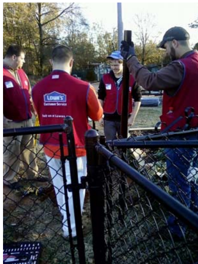
Lowe's Heroes Workers Install Fence around Raised Garden Beds
